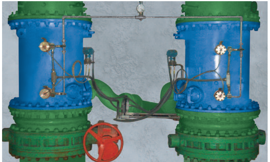
PR-BW 800-C filter in a power plant
